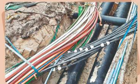
Under Ground Electrification
